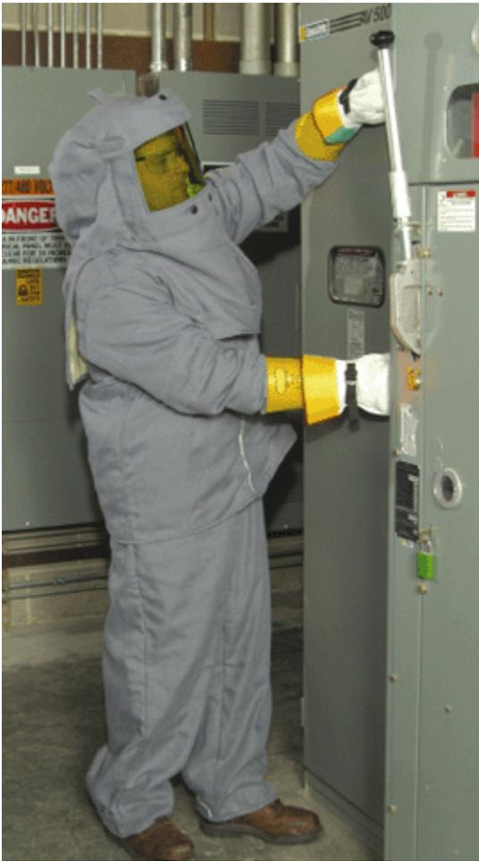
*In order to know the appropriate level of personal protective equipment, it is necessary to analyze the hazard at each panel or piece of equipment. Each analysis starts by knowing the available fault current at that location.*
