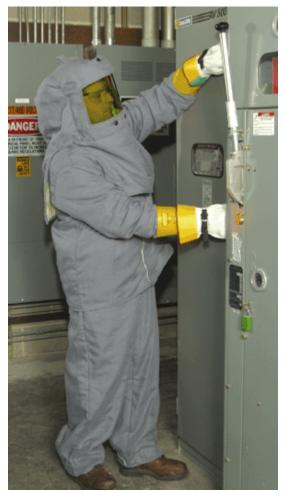
In order to know the appropriate level of personal protective equipment, it is necessary to analyze the hazard at each panel or piece of equipment. Each analysis starts by knowing the available fault current at that location.
